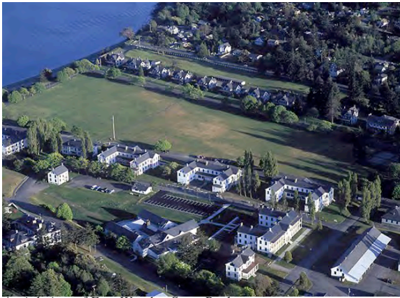
Aerial view of Fort Worden State Park [Photo Courtesy Centrum Music and Performance Center]
