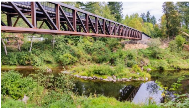
A new bridge spans the Chehalis River between Dryad and Doty
