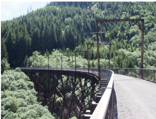
West of the Cascades the trail uses several former railroad trestles
